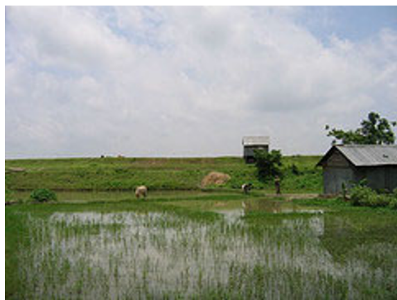
Figure 1 View of the MDIP embankment from a bari located inside of the flood protected area.
